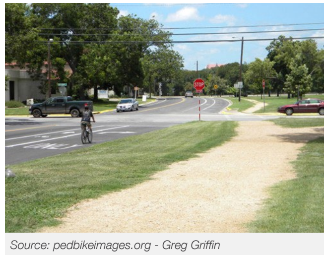
Figure 5-9. All-Way Stop-Controlled Intersection Example
