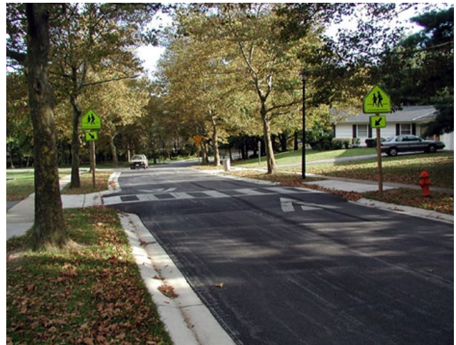
Figure 5-12. High-Visibility Crosswalk Example
