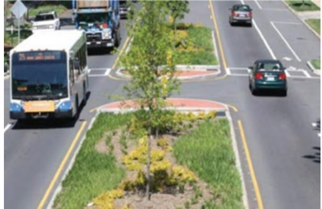
Figure 5-3. Raised Median Example
