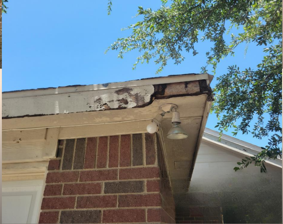
Damage fascia – Exposed framing
