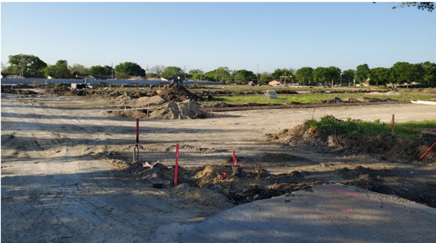
72,000 square-foot Flex Office Space under construction at 3500 IH-30
