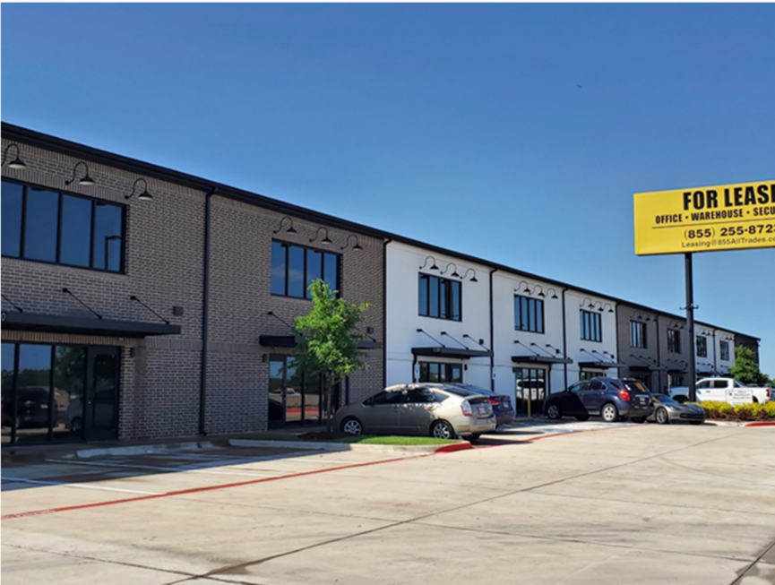
AllTrades WorkSpace Shops and Studios 2828 IH-30
