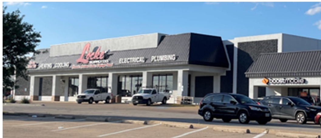
Locke Supply - 34,000 square-foot Reuse of vacant Minyard Food Store Oates Park Shopping Center
