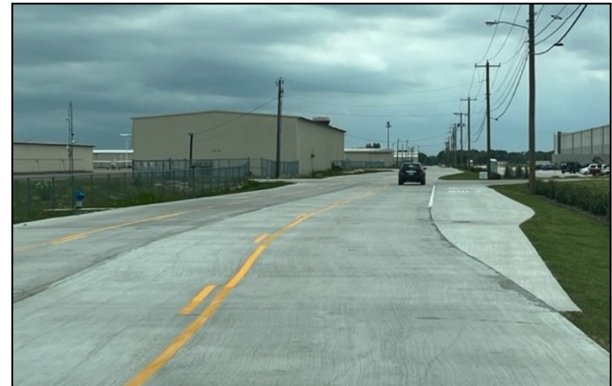
Airport Boulevard Reconstructed
