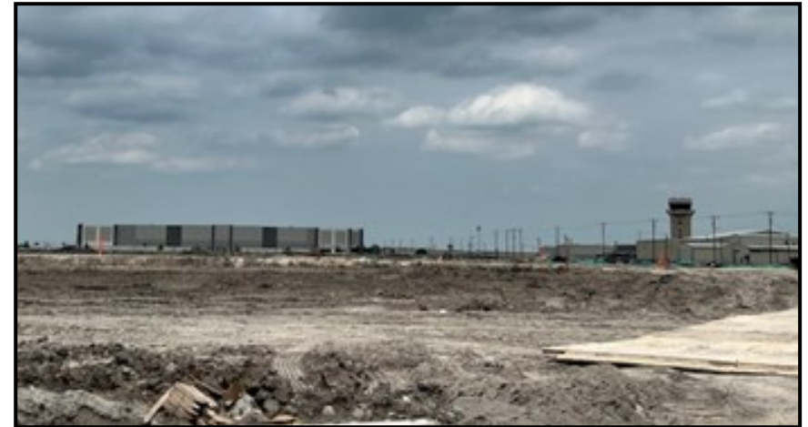
Phase 2 Under Construction
