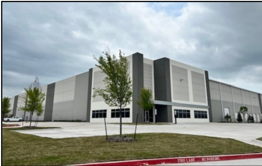
Phase 1 - Building 1 Completed
