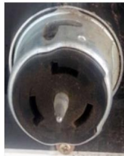
120/240 Volt, 50 Amps, Twist Lock – 3 Wire
