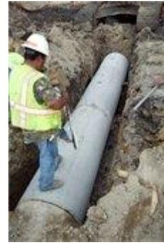
**What's happening now:** The contractor has placed main lines under all southbound lanes and has begun the installation of storm sewer and waterline extensions across the northbound lanes. Contractors are concurrently repairing sidewalk connection from Motley to Rustown Drive.
