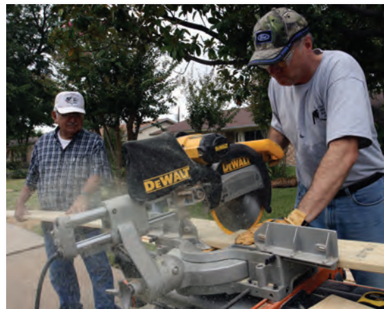
Assistant City Manager Jerry Dittman saws wood for new wheelchair ramp.
