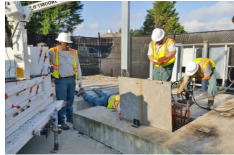
City of Mesquite Employees perform repairs to City's facility.
