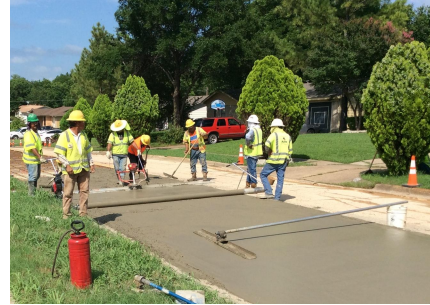
City of Mesquite Employees perform repairs to a City street.
